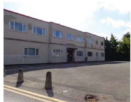
Industrial Works along St. Hilda's Street
