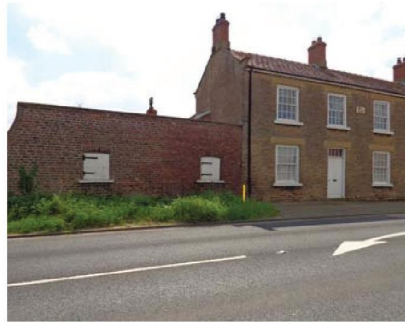
Manor Farm and wall along the A64
